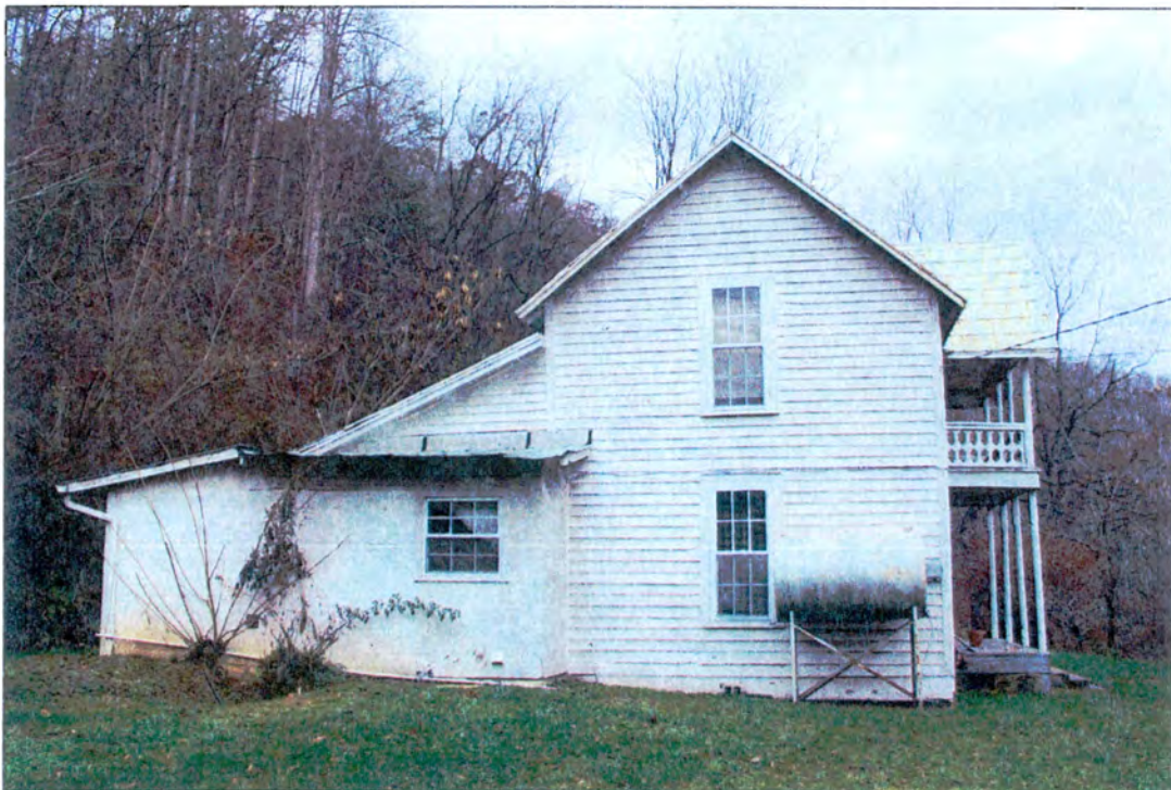
Photo 4: East side elevation with concrete block additions.
