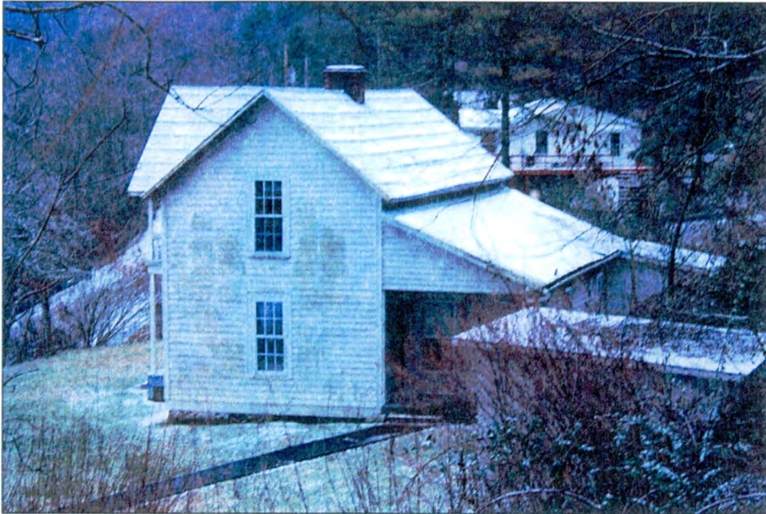
Photo 3: West side and south rear elevations.
