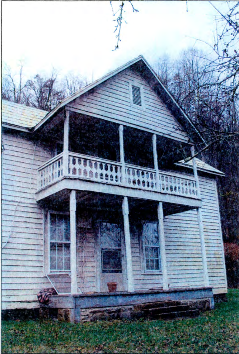
Photo 5: North elevation showing two-story portico and compacted fenestration.
